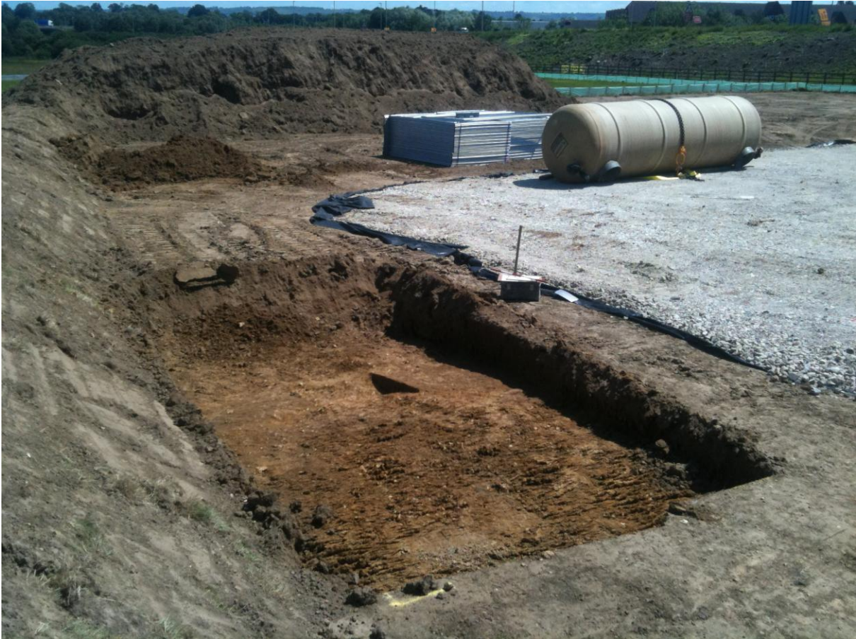
Figure 2 Ditch revealed during excavations associated with proposed septic tank (note the depth of surviving topsoil and subsoil).
