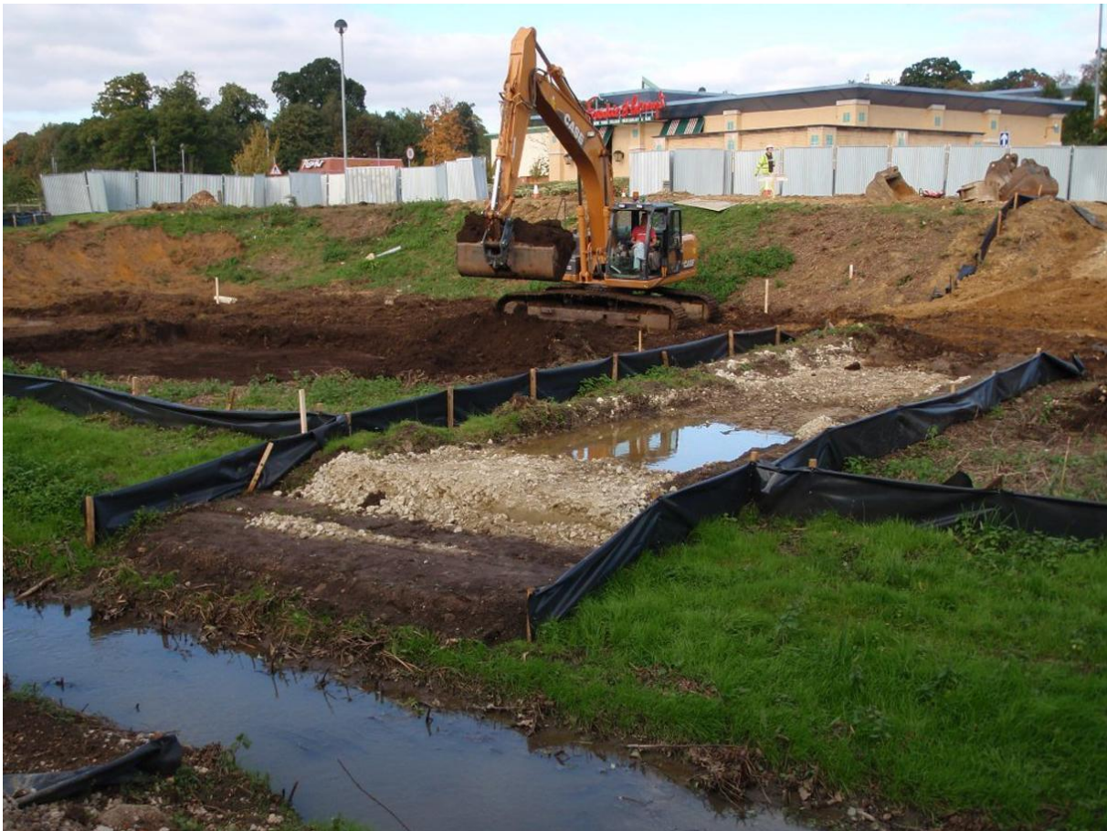
Plate 1 Removal of topsoil with northern extent of proposed footbridge
