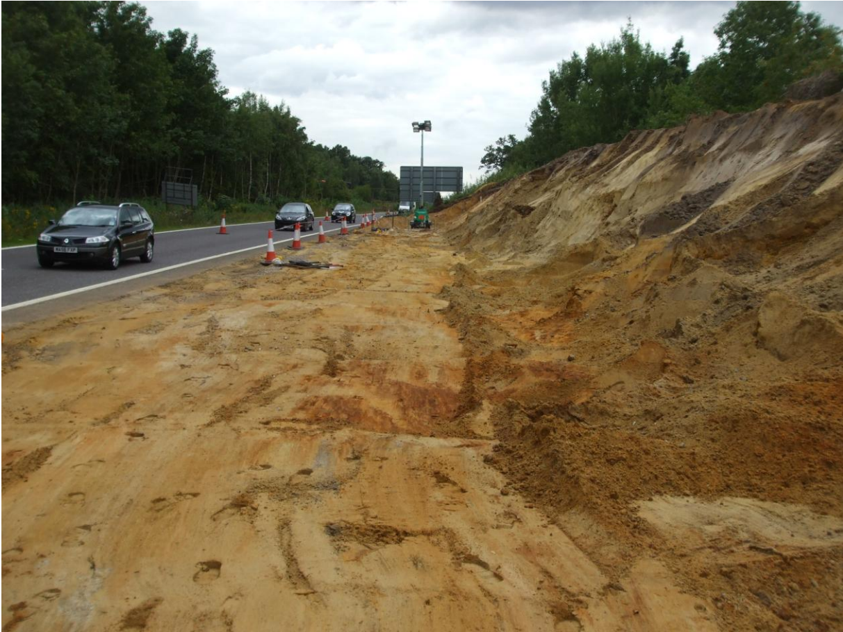
Plate 2 Made ground within Area 8 looking up M20 slip road
