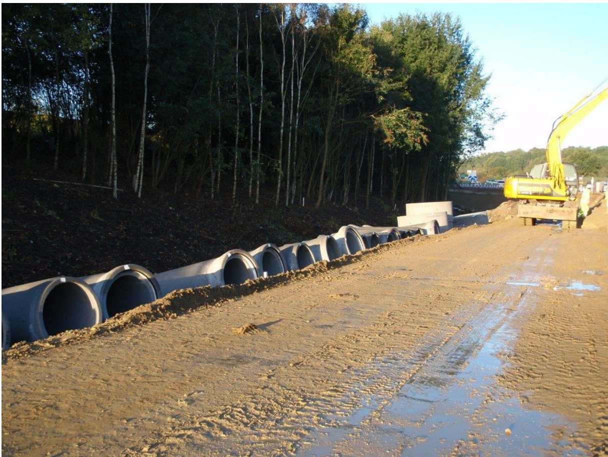
Plate 1 Imported Type 1 stone (shown) directly overlay made ground within Area 8
